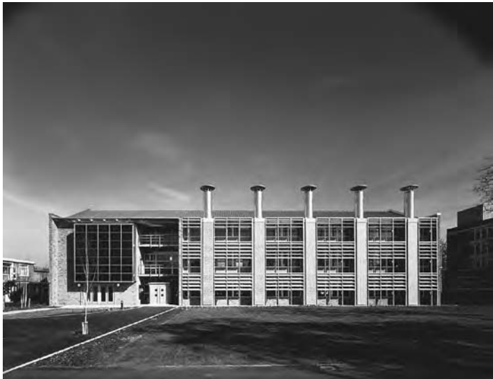
14.1 South façade of the building.
