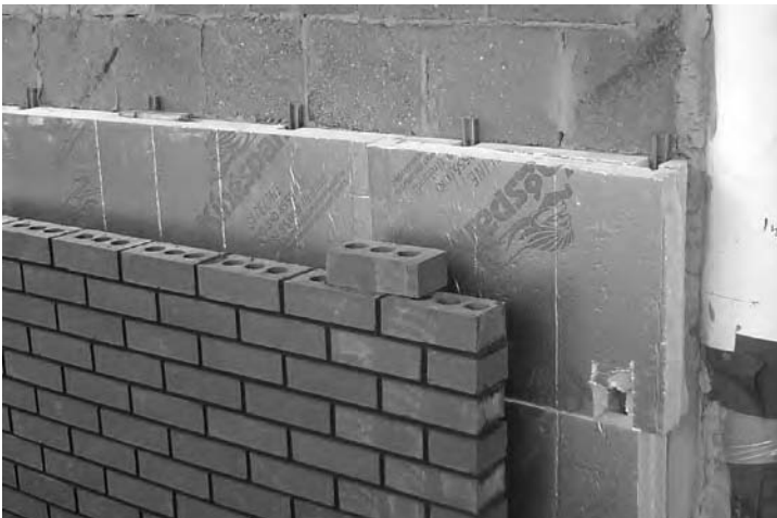
B.1 The wall under construction.
