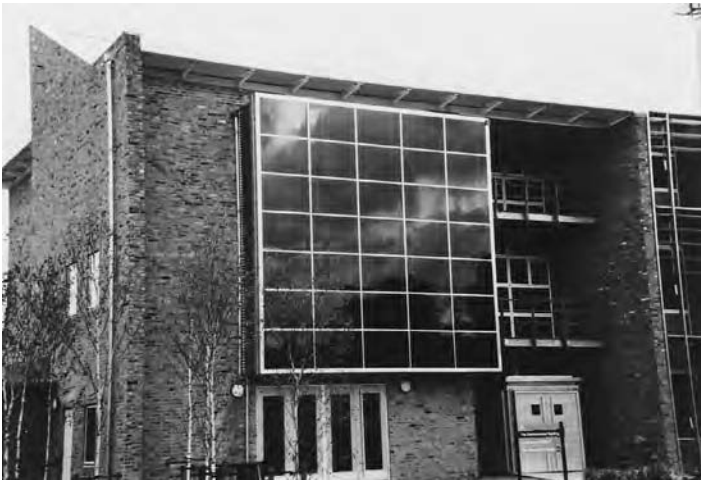
14.10 PV panels on the south façade.
