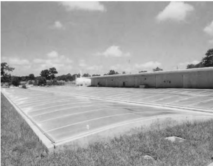
7.4 Solar water heating at a Florida alligator farm. 15
